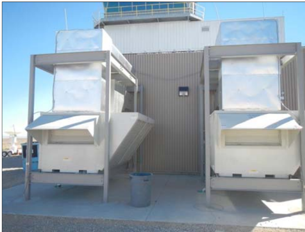
SNL Tonopah Main Distribution Hub
