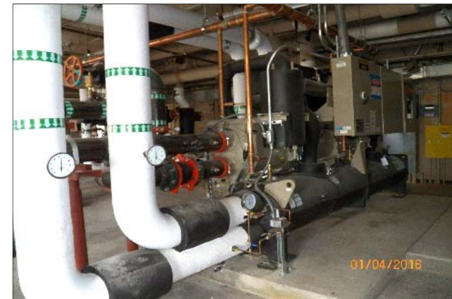
LLNL B131 Chiller Replacement
