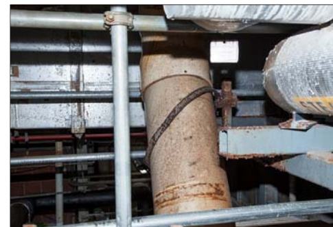
Y-12 Kathabar System Failure
