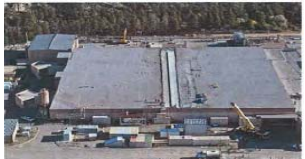
New Drag Strut across PF-4 Roof
