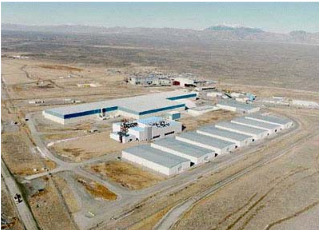
Advanced Mixed Waste Treatment Project, Idaho National Laboratory
