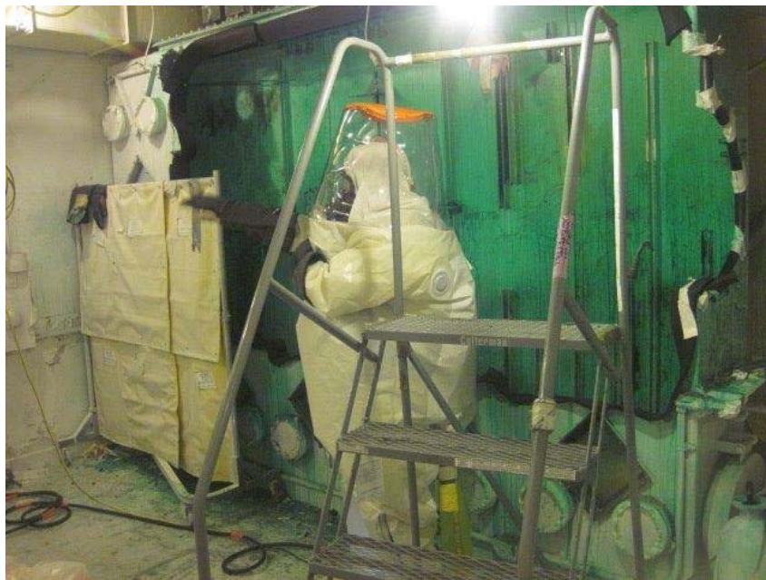
Glovebox Dismantlement in the Hanford Plutonium Finishing Plant
