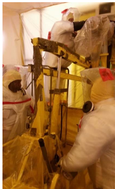
Mock-up Training for Building 235-F Remediation
