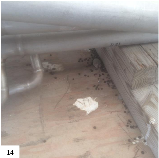
Figures A-11 to A-14. Staff review team photographs illustrating deficient storage tents. Figure A-11 shows a ripped tent at the MHF Laydown Yard. Figures A-12 and A-13 show ripped tents at the Waste Treatment and Immobilization Plant (WTP) construction site. Figure A-14 shows evidence of animal intrusion in a tent at the WTP construction site.
