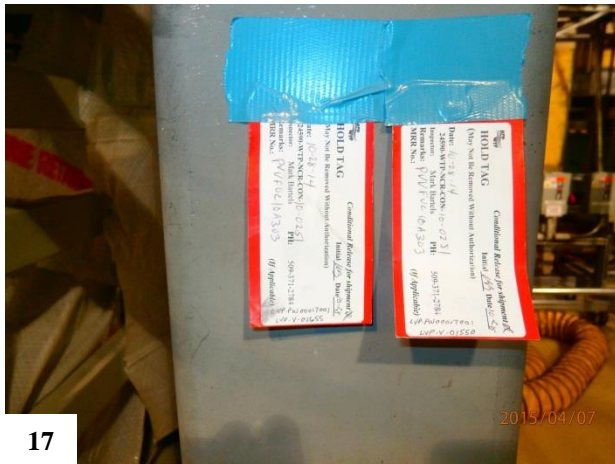
Figures A-15 to A-18. Staff review team photographs illustrating alternate methods of identifying nonconforming items. Figures A-15 to A-17 depict Nonconformance report (NCR) hold tags on structural steel near the nonconforming item. Figure A-18 shows NCR hold tags on the outside of a storage tent near the Pretreatment Facility construction site.
