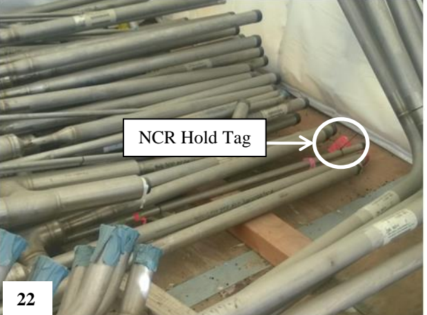
Figures A-19 to A-22. Staff review team photographs illustrating nonconforming SSCs that were not properly segregated. Figures A-19 and A-21 are inside the High-Level Waste Facility. Figure A-20 was inside a storage area at the WTP construction site. Figure A-22 was inside a storage tent near the Pretreatment Facility.
