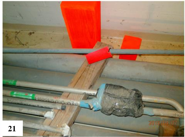
Figures A-19 to A-22. Staff review team photographs illustrating nonconforming SSCs that were not properly segregated. Figures A-19 and A-21 are inside the High-Level Waste Facility. Figure A-20 was inside a storage area at the WTP construction site. Figure A-22 was inside a storage tent near the Pretreatment Facility.
