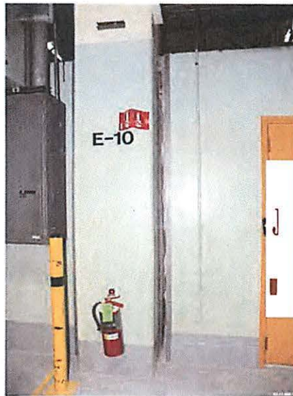
Figure 2. Captured Column in Plenum Room (Wall Cut Back 1.5 in.)
