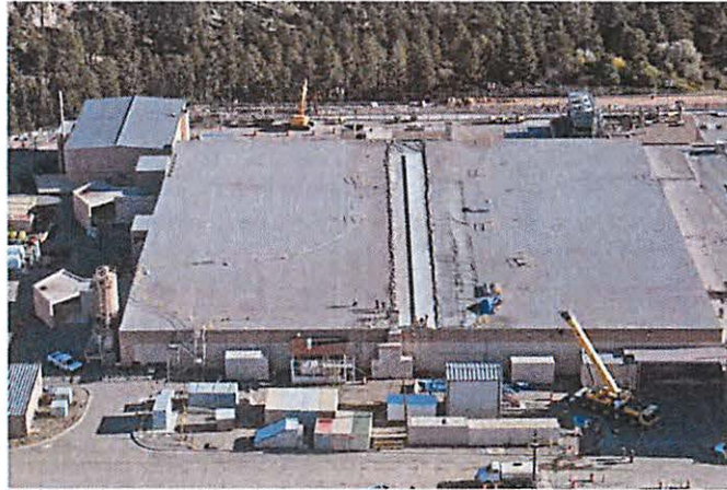
Figure 1. New Drag Strut Across PF-4 Roof
