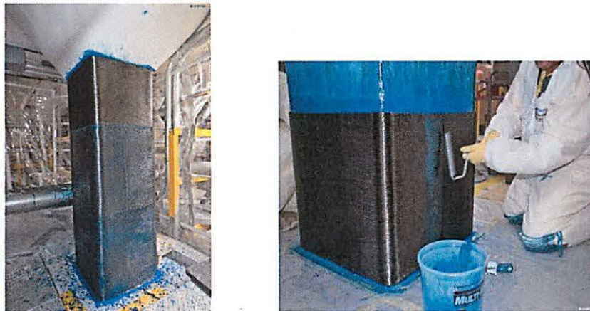
Figure 5. Basement Column reinforcement
