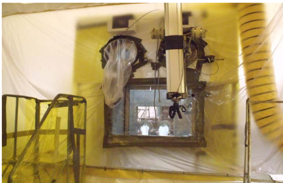
Building 235-F Cell Mock Up for Deactivation Containment Work
