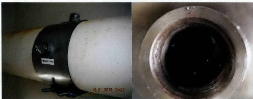
Figure 2: Typical Flow Test Port
