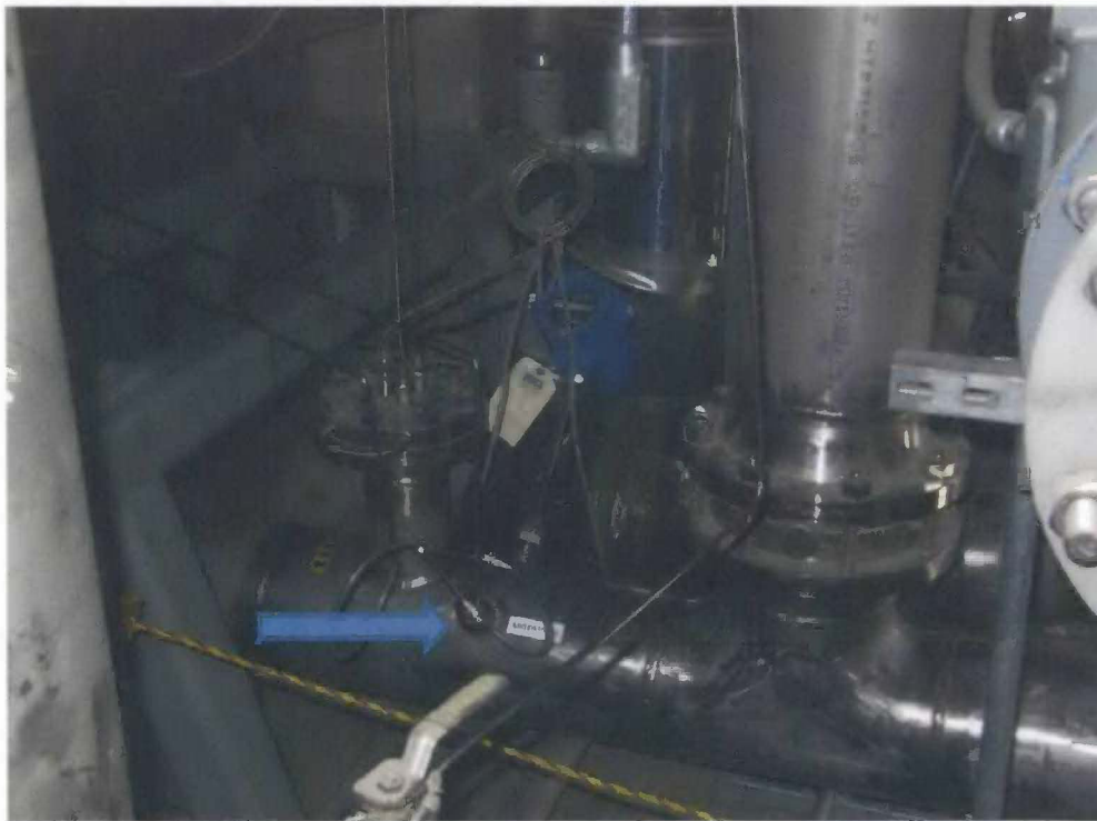
Figure 4: AZ-102 Flow Test Ports
