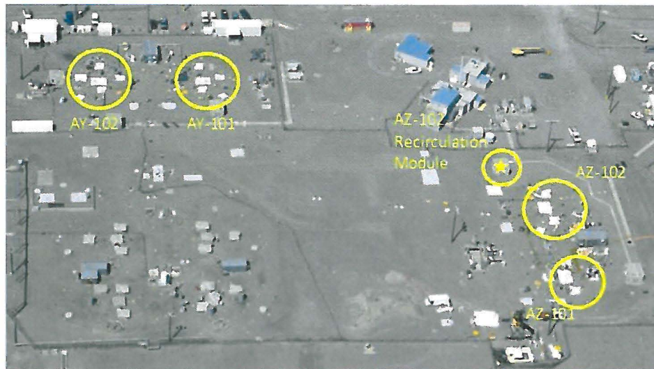
Figure 1. AY/AZ Tank Farm.
