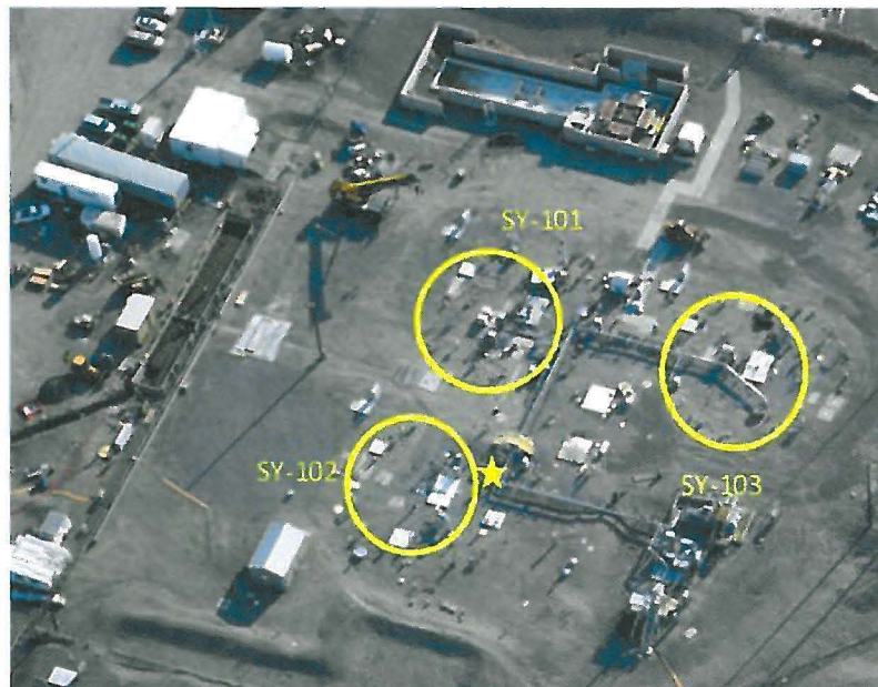
Figure 2. SY Tank Farm.
