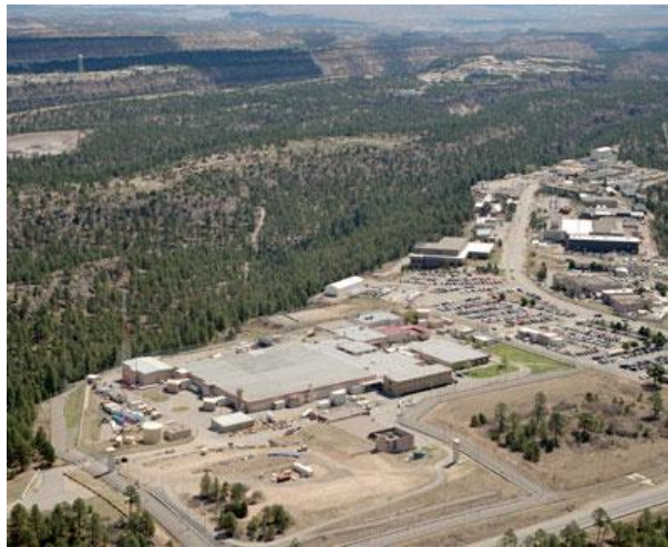
Plutonium Facility (PF-4, in foreground)
