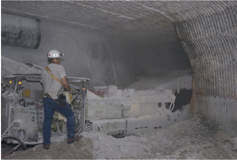
Mining Operations at the Waste Isolation Pilot Plant
