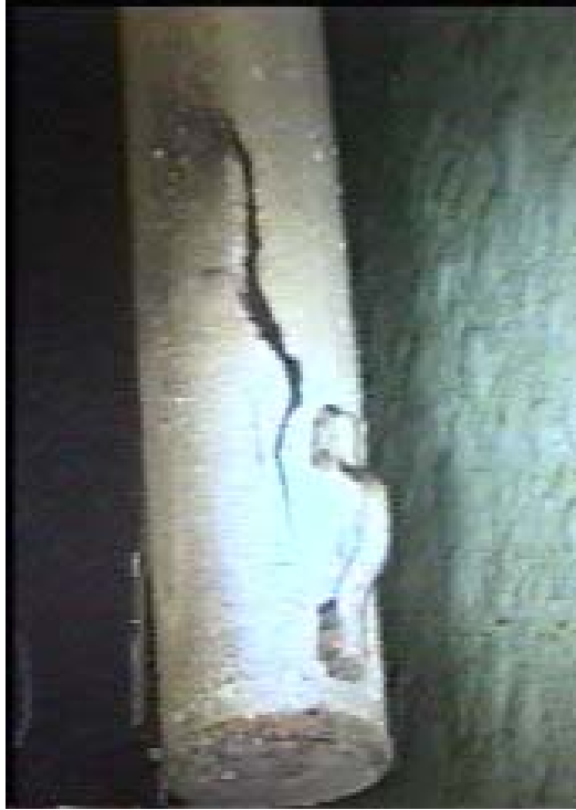
Figure 3. Lower portion of a cracked Z can.
