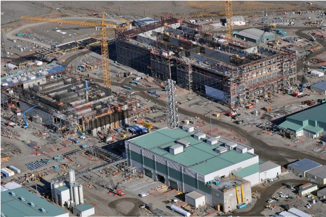
Construction Site, Waste Treatment and Immobilization Plant
