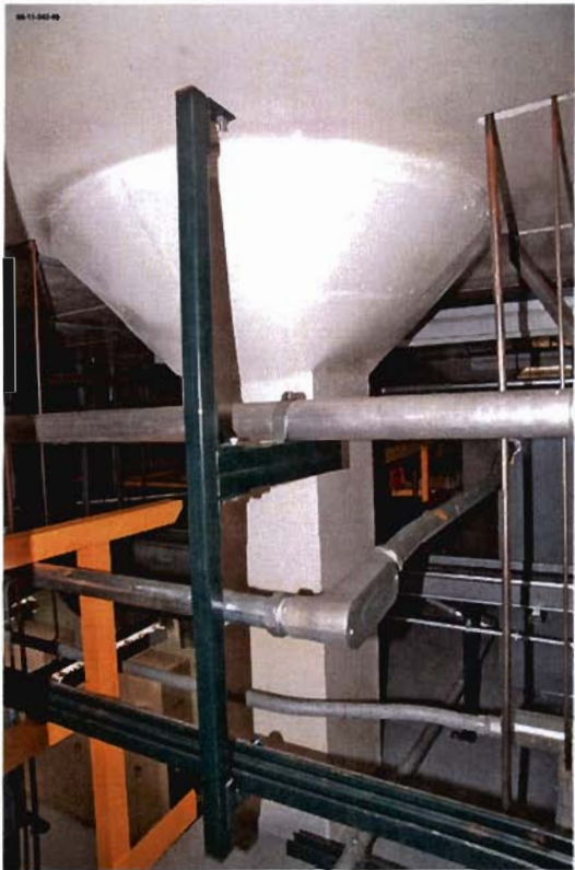
Figure 8. Vault Captured Column
