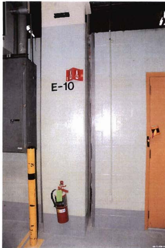
Figure 4. Captured Column in Zone 1 Plenum Room (Wall Cut Back 1.5 in.)
