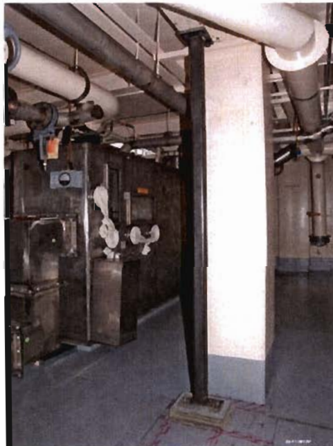
Figure 1. New Steel Column Supporting Steel Beam
