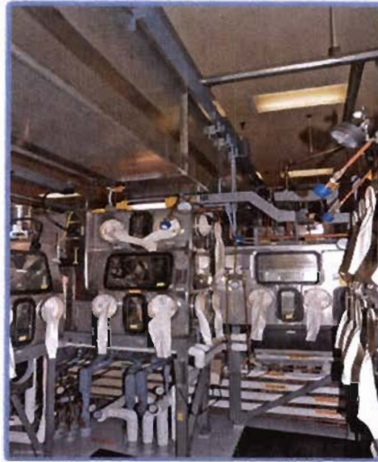
Figure 11. Glovebox Support Stand (Gray) and Glovebox Services
