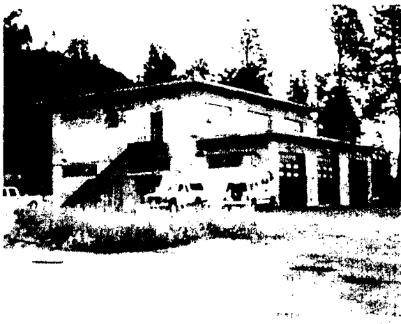
Fire Station 5 (TA-16-180)
