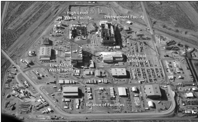
2007 saw significant construction progress in the facilities not affected by the seismic design criteria
