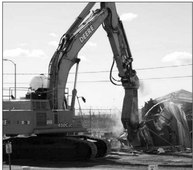
Demolition of 241Z
