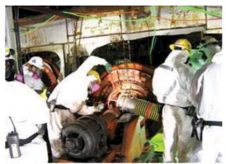
High Risk Equipment Compressor Seal Exhaust Lines are Cut and Isolated
