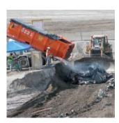
Contaminated Soil and Other Material from Hanford's River Corridor Is Being Disposed of in the Environmental **Restoration Disposal** Facility. Water Is Being Applied for Dust Control
