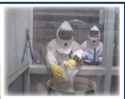
Consolidated Radioactive Sludge (an Estimated 55 Cubic Yards) Vacuumed from the Floors of Hanford's K East Basin. Began Transferring the Sludge Out of the Basin in Preparation For Draining and Removing the Leak-Prone Pool
