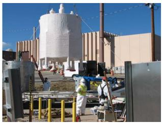
Workers Remove the 20+ Year-Old Caustic Tank at TA-50 Rad Liquid Waste Treatment Facility
