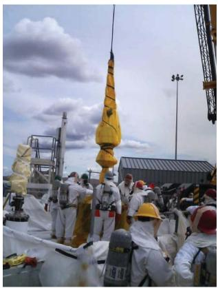
Removing a Failed Sluicer at Tank C-103
