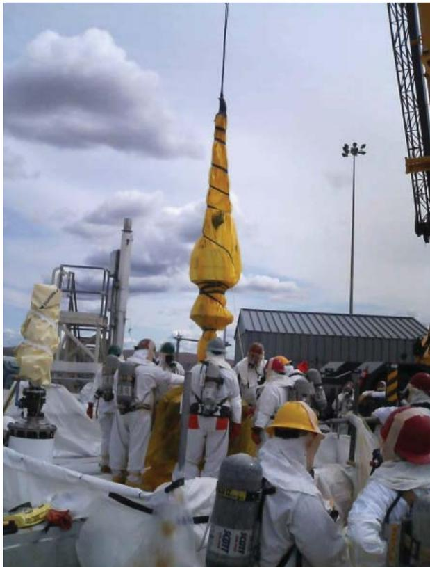
Removing a Failed Slucicer at Tank C-103
