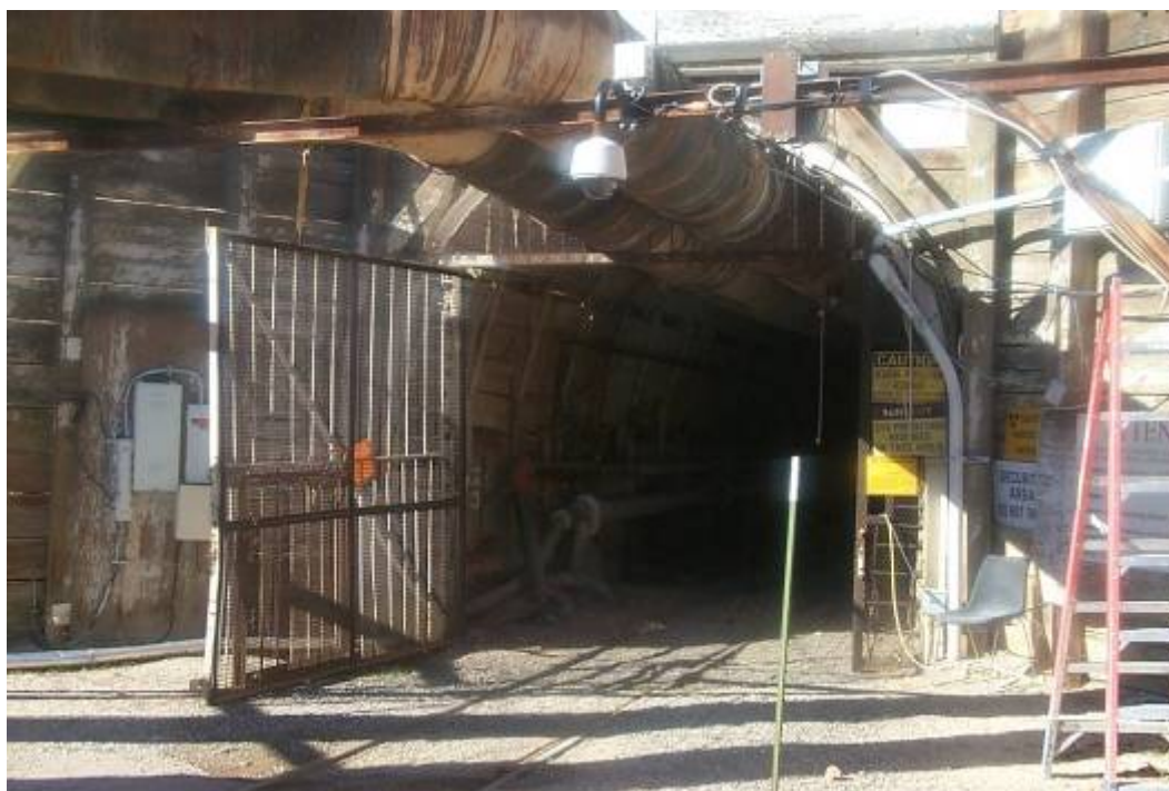
Figure 4-6. First 200 feet of timber scheduled for fire retardant coating.
