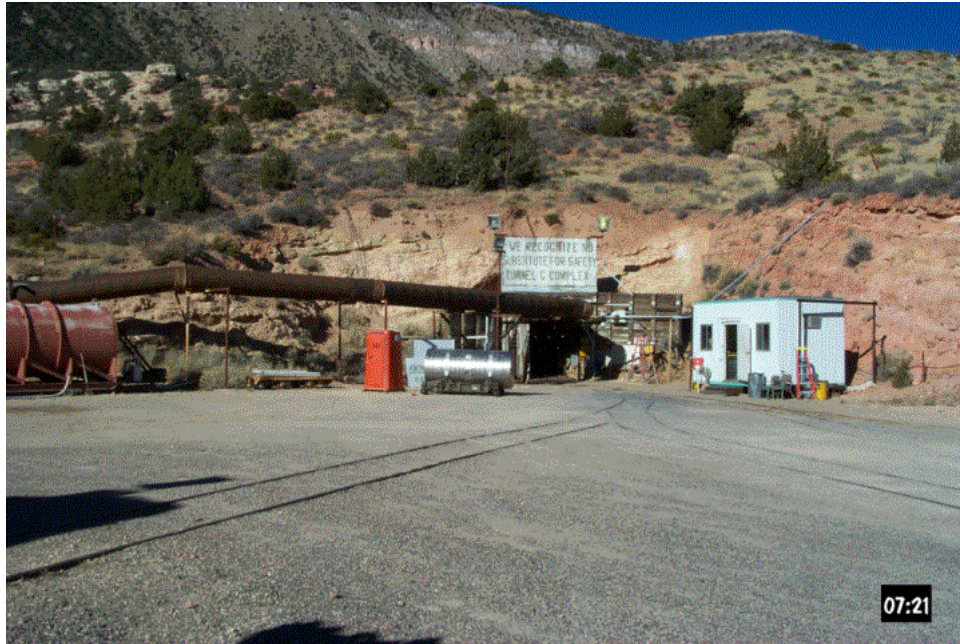
Figure 2-1. U12g Tunnel portal entrance.
