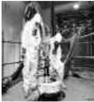
**WORKERS USING PNEUMATIC AND MECHANICAL RETRIEVAL SYSTEMS TO REMOVE WASTE FROM THE SILO AND PACKAGE IT IN SOFT-SIDED CONTAINERS FOR OFF-SITE SHIPMENT.**
