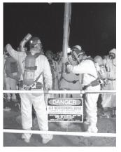
Hanford Tank Farm workers installing a breather stack extension.
