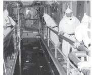
Team members of the K Basins Decontamination and Decommissioning project begin pouring grout to permanently fill and secure the discharge chute.
