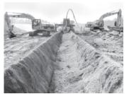
Hydrologic isolation activities for Solid Waste Storage. This includes employing a state-of-the-art trenching technology that ensures that the project meets the regulatory requirements for reducing groundwater infiltration into the Waste Burial Grounds at Y-12.
