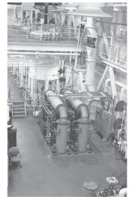
Lawrence Livermore National Laboratory Decontamination and Waste Treatment Facility use evaporators to remove Radioactive and Hazardous Solids from Wastewater.
