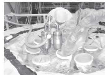
*Workers at the Sludge Retrieval and Disposition Project connect hoses to ports in the top of large diameter containers that will hold sludge from the North Loadout Pit in the K East Basin at the Hanford Site.*
