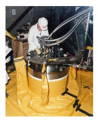
**Cover Photograph:** Nuclear Chemical Operators Attach Hoses to Ports in the Top of a Multi-Canister Overpack Holding 290-300 Irradiated Fuel Assemblies from Hanford's K-Basins, in the Cold Vacuum Drying Facility.
